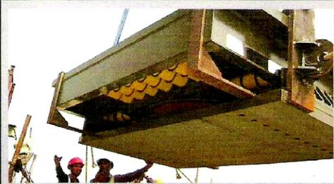
**EradiQuake® Seismic Isolation Bearings by mageba\***
